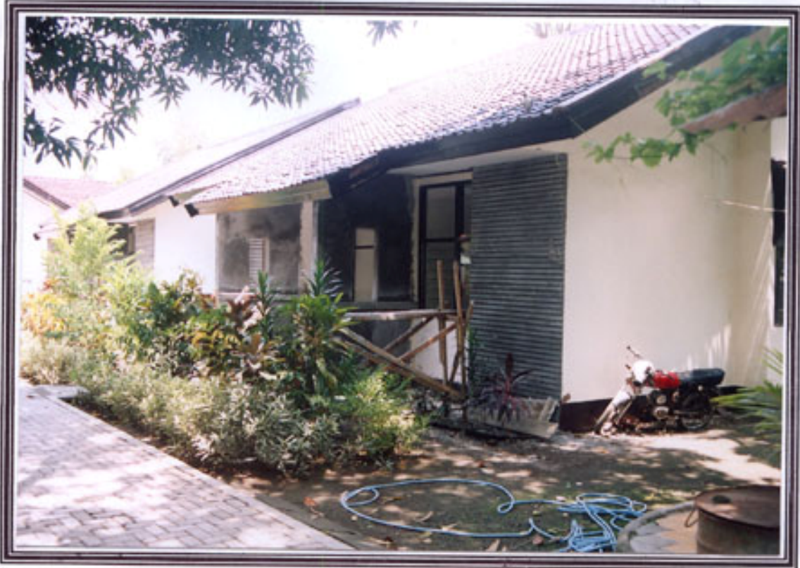
RENOVASI WISMA ( TAMPAK SAMPING )
